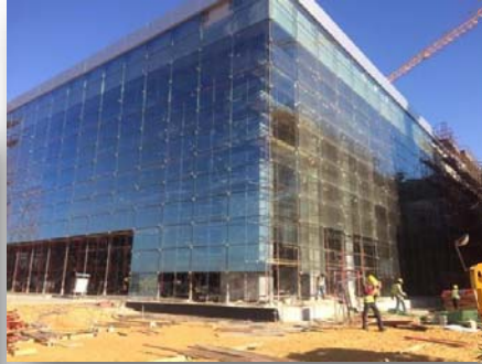
2- The New Opera House (New capital)
